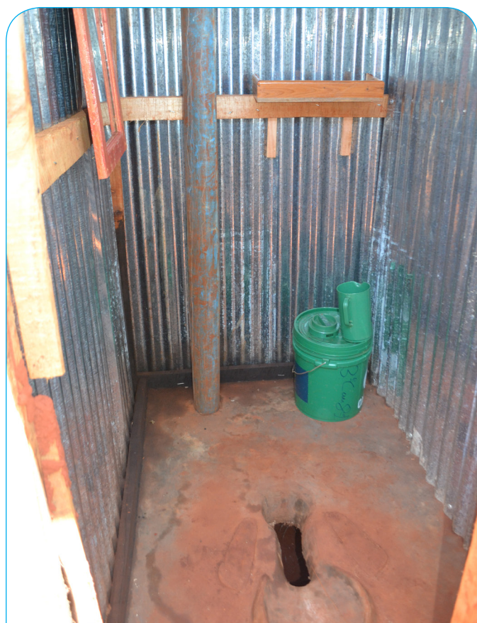
A sample of a female toilet in a school in Nyaragusu Camp including a water source, mirror, shelf and hook for hygienically storing menstrual materials and supplies while in use. © Columbia University; International Rescue Committee.
