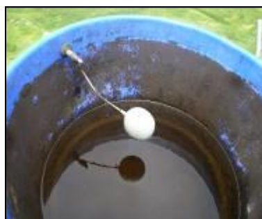
UNICEF Colombia: water storage tank
